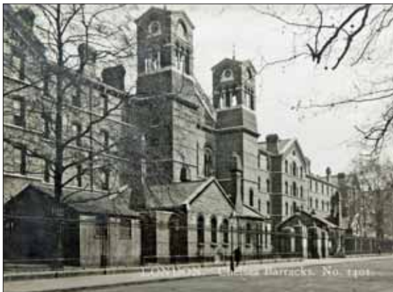
A Postcard view along Chelsea Bridge road in the 1900's. The Tower on the left of the main entrance had a large clock with faces on the road and barrack square side whereas the tower on the right had two faces that showed wind direction. The building in the foreground, at left, was constructed around 1897 and became the Commanding Officer's office and Sergeant Major's office matching the building opposite which was the Guard Room and was provided at the time of opening.
