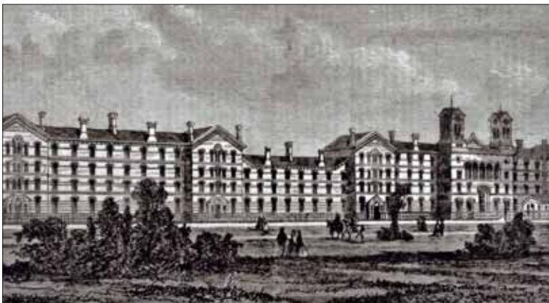
A view of Chelsea Barracks that appeared in the Illustrated London News in December 1861. The Stepped roof line was levelled in 1897 by adding floors either side of the central section following a fire that destroyed part of the upper floor in A Block, the nearer one of the left.
